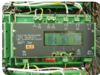
The LCD display shows the data points sent to a controller via network communication. The LEDs show proper network activity..
