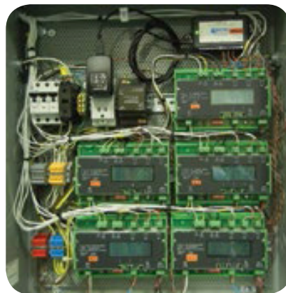
Five APN monitors monitoring the AC units at NK Technologies' factory in San Jose, CA..
